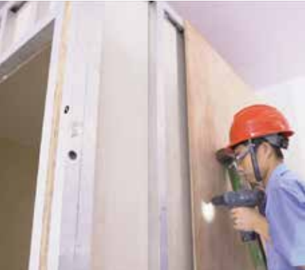
Clapboard installation by third party(FC board available)
