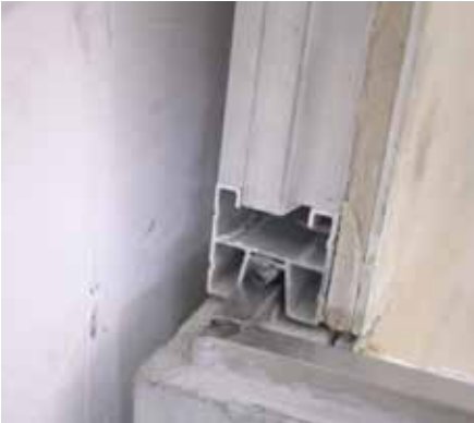
Gap between wall and base sealing
