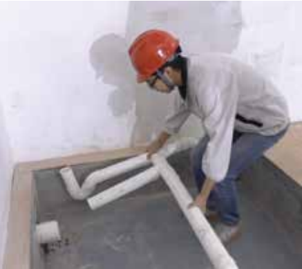
Prefabricated drains installation
