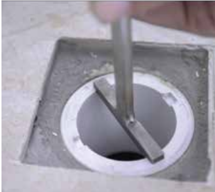
Sally waterproof flange installation
